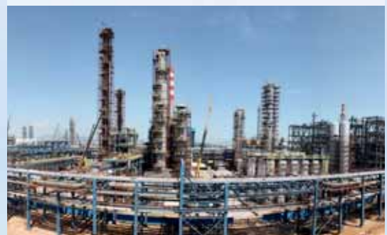
Power Generation Industry
